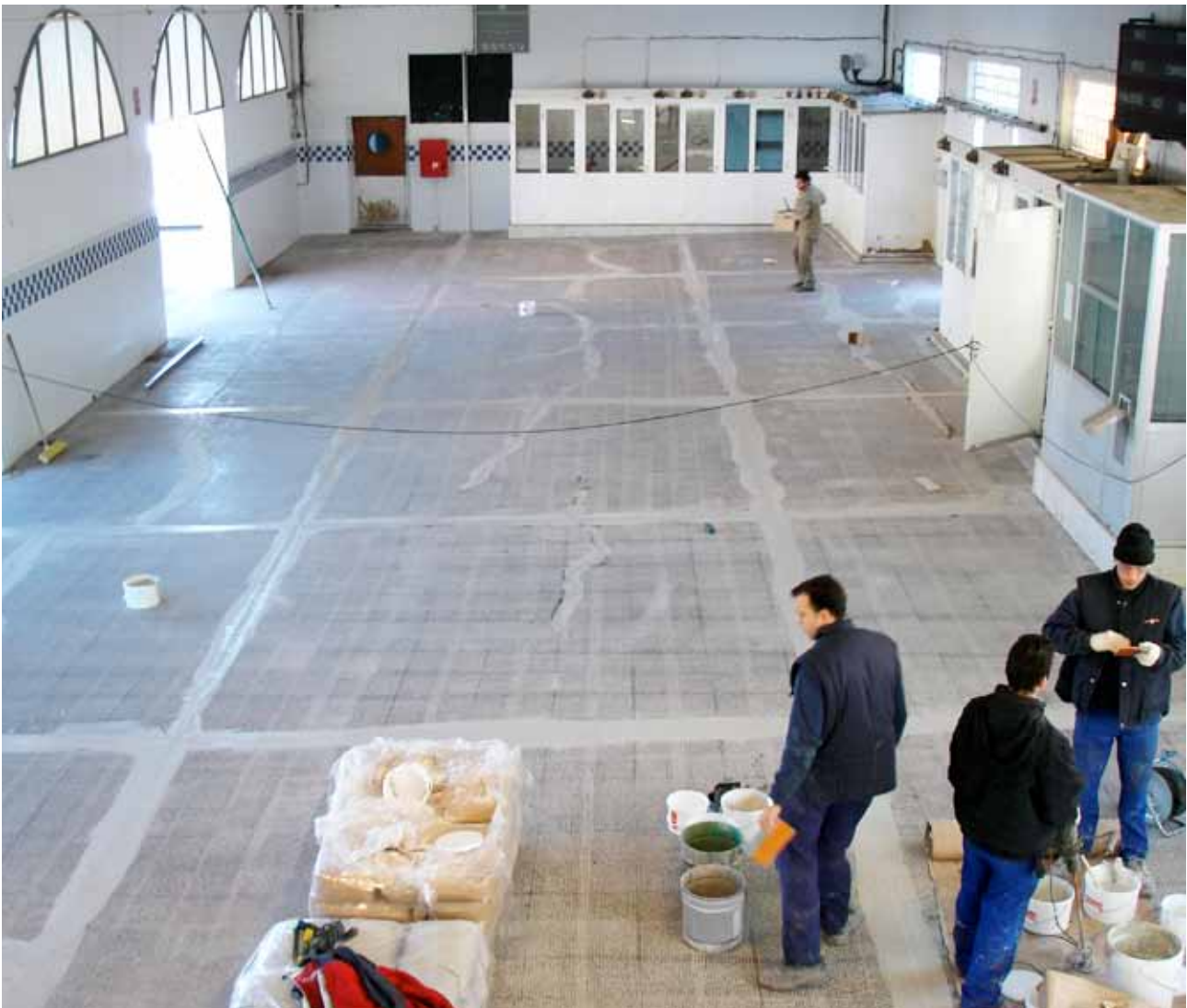
Floor support after preparation and treatment of rupture joints with resin and sand, as a dry mortar
