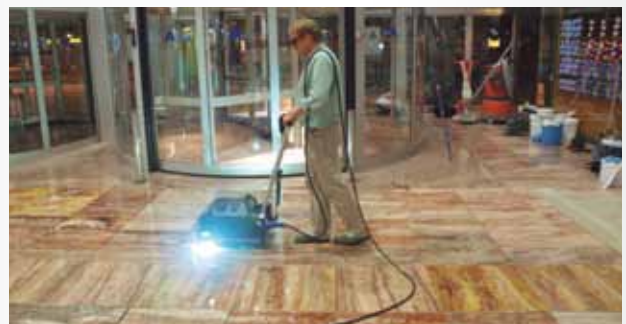
Curing the resin by UV machine, drying instantly
