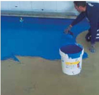
Top coat application, coloured sealing
