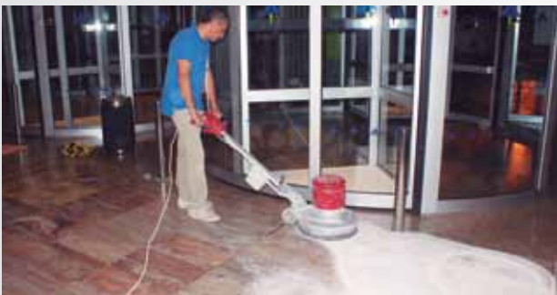
Prepare floor with a sanding disc machine, in order to open the pores in the pavement and improve penetration and mechanical adhesion of the system.
