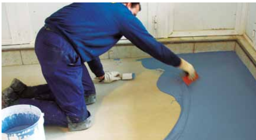
Application of base coat
