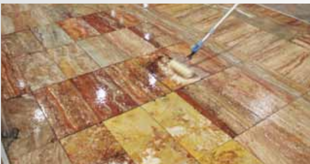
Application of the UV resin
